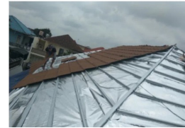
Gambar 1.2 Peredam Panas Aluminium Foil
